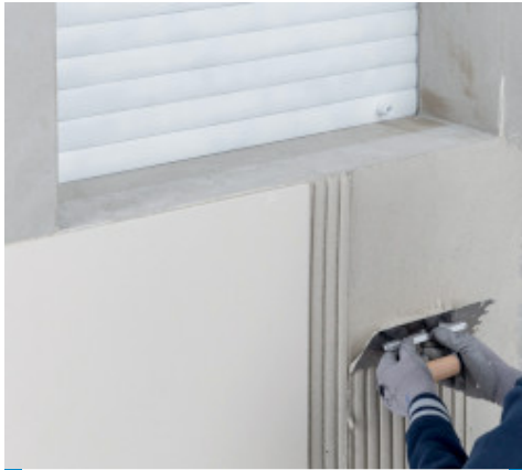
Installation of large-size ceramic tiles
