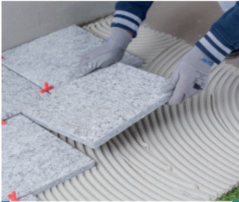
Installation of natural stone in exterior
